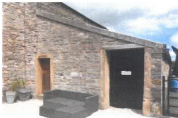
Photograph (9) – South lean –to return elevation
