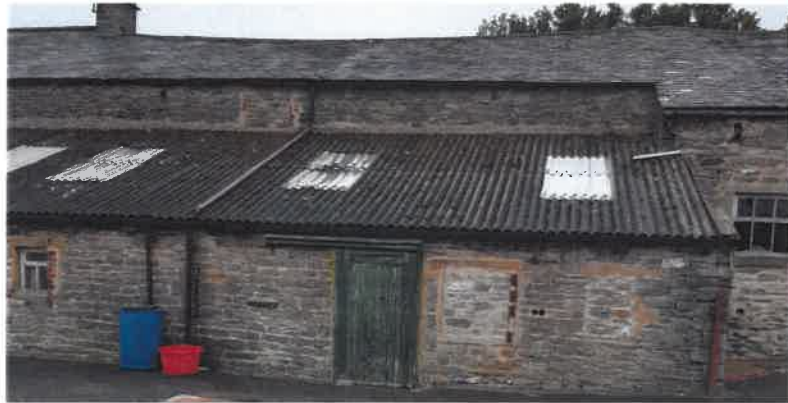
Photograph (6 & 7) – South elevation
