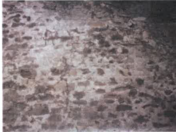
Photography (10) – Internal wall
