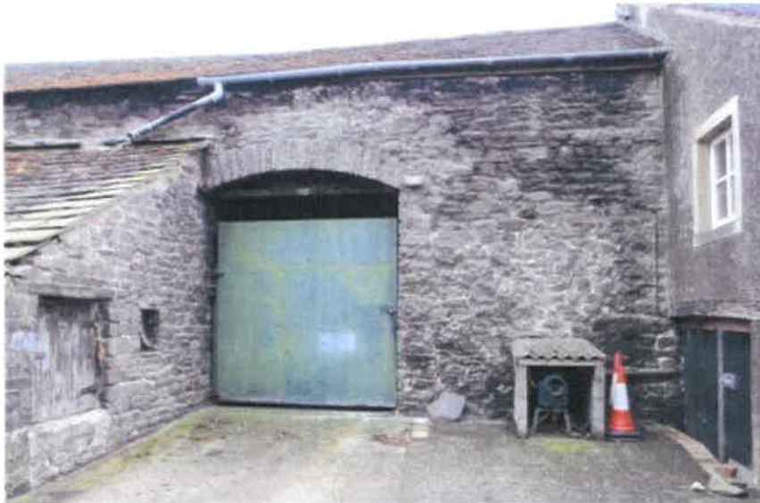
Photograph (5) Lean -to Return and cart opening
