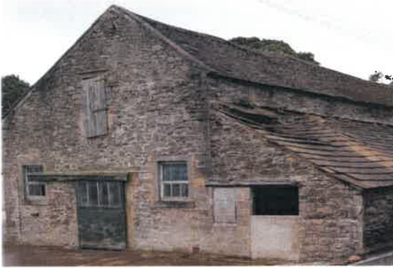
Photograph (3) – East elevation
